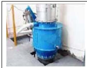
*The picture shows a Discharge Valve (In Blue) with a Temporary Storage Chamber above it.*
